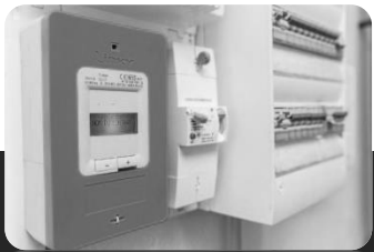
PRE-FIXATION OF ELECTRICAL BOX
